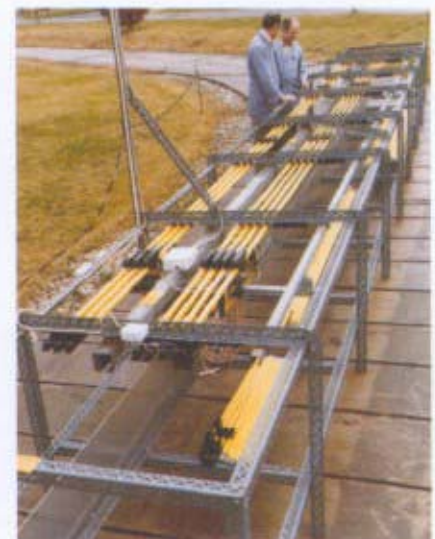
Test installation at SIEMENS for the transmission of data and telephone signals.
